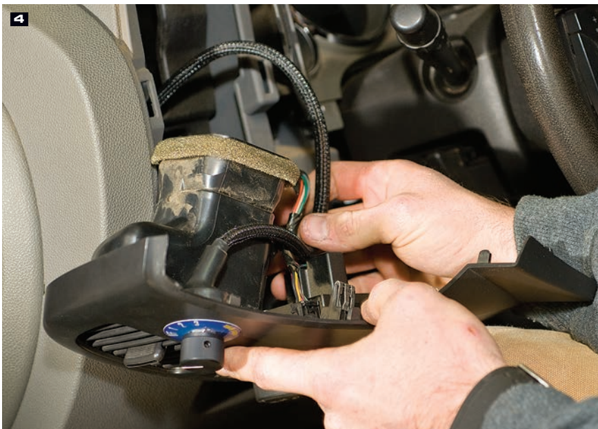
4) Lock the BD control switch in place and then replace the panel.
