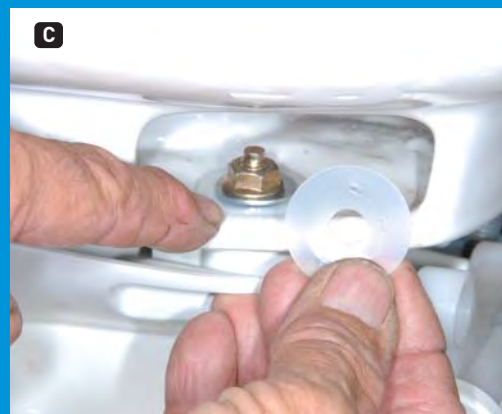
A) New waste ball seal is positioned with the flat side down. B) The bowl is then placed back on the plastic base and new washers are used before loosely tightening the nuts. C) New flange seal is positioned before the toilet is placed back on the floor.
