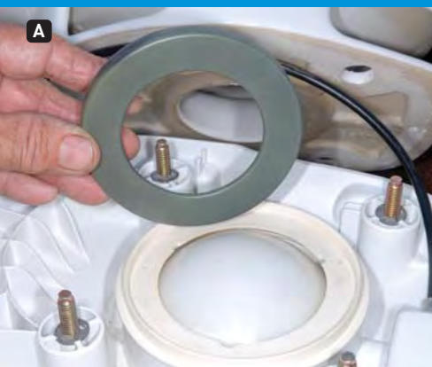
A) New waste ball seal is positioned with the flat side down. B) The bowl is then placed back on the plastic base and new washers are used before loosely tightening the nuts. C) New flange seal is positioned before the toilet is placed back on the floor.
