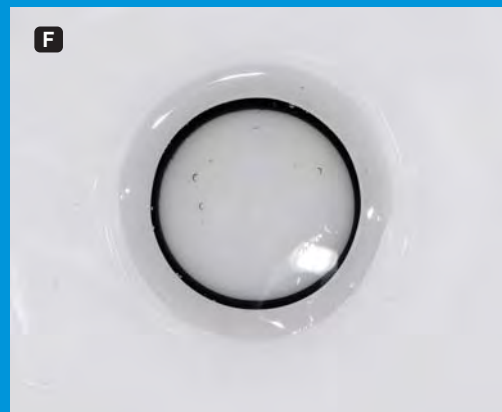
D) Before final tightening of the bowl to the base, the waste ball seal here needs to be centered. E) This can be accomplished by opening the toilet seat and lifting the bowl from the base and gently centering the seal. The nuts are then tightened. F) Nuts holding toilet to the closet flange are tightened before the water line is reconnected.
