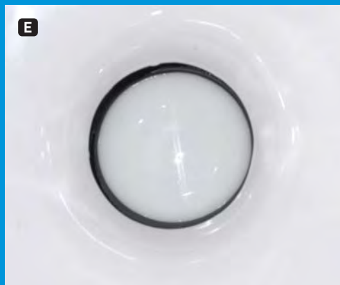
D) Before final tightening of the bowl to the base, the waste ball seal here needs to be centered. E) This can be accomplished by opening the toilet seat and lifting the bowl from the base and gently centering the seal. The nuts are then tightened. F) Nuts holding toilet to the closet flange are tightened before the water line is reconnected.
