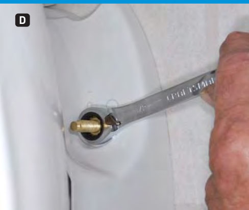
D) Before final tightening of the bowl to the base, the waste ball seal here needs to be centered. E) This can be accomplished by opening the toilet seat and lifting the bowl from the base and gently centering the seal. The nuts are then tightened. F) Nuts holding toilet to the closet flange are tightened before the water line is reconnected.
