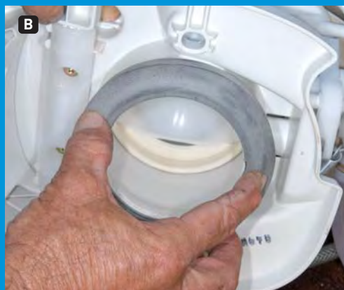
A) New waste ball seal is positioned with the flat side down. B) The bowl is then placed back on the plastic base and new washers are used before loosely tightening the nuts. C) New flange seal is positioned before the toilet is placed back on the floor.
