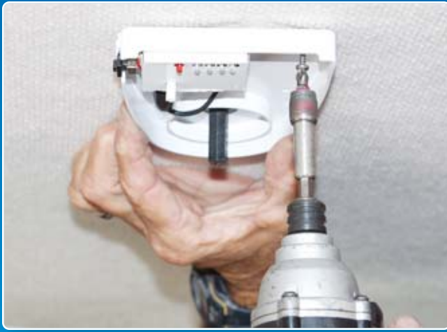
Attach the enclosure base to the ceiling of the trailer with supplied screws.
