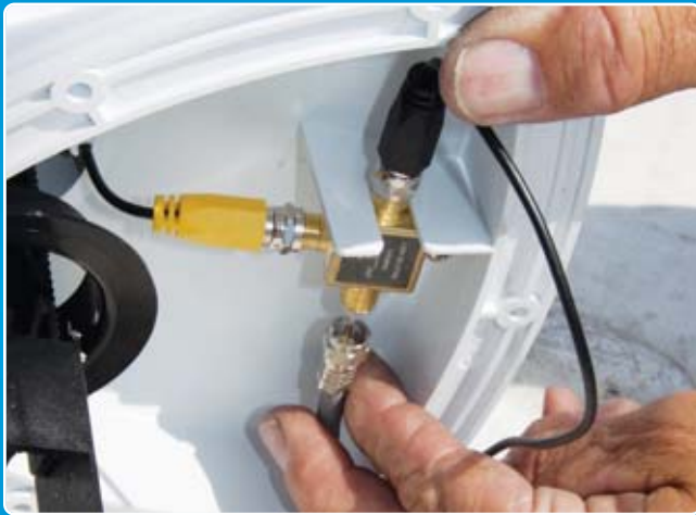
Use the existing coax cable from the old antenna and attach it to the T-connector.
