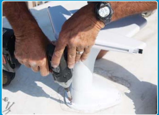
Set the antenna into place with screws that are the proper length (not supplied).
