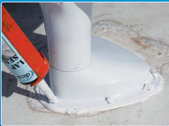
Apply the appropriate type of sealant around the base and over the screw heads.
