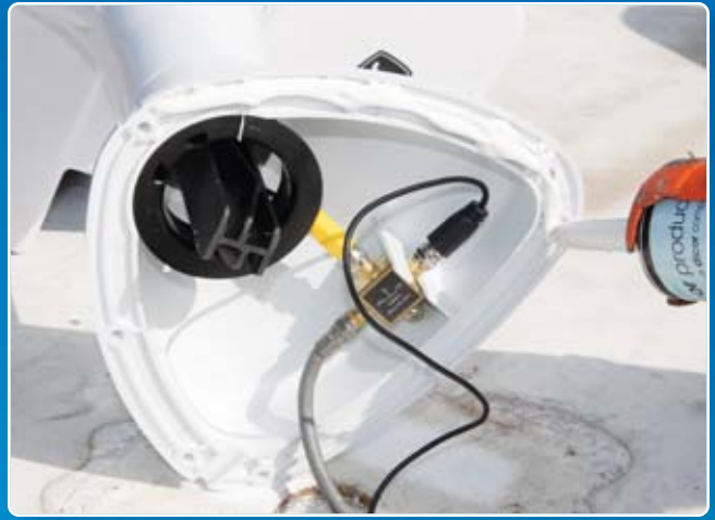
Apply sealant to the bottom of the flange on the base mount and the ring seal. Butyl tape may also be used where applicable.
