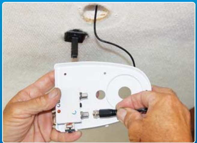
Attach the coax from the upper unit to the SureLock signal meter's enclosure base.
