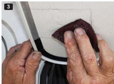
1) Measure 4 inches from the top edge of the door for the leading edge of the mounting plate. 2) With the mounting plate held into position, pencil a line around the outside edge. 3) Using the scuff pad, rough up the outlined area for the first step of prep.
