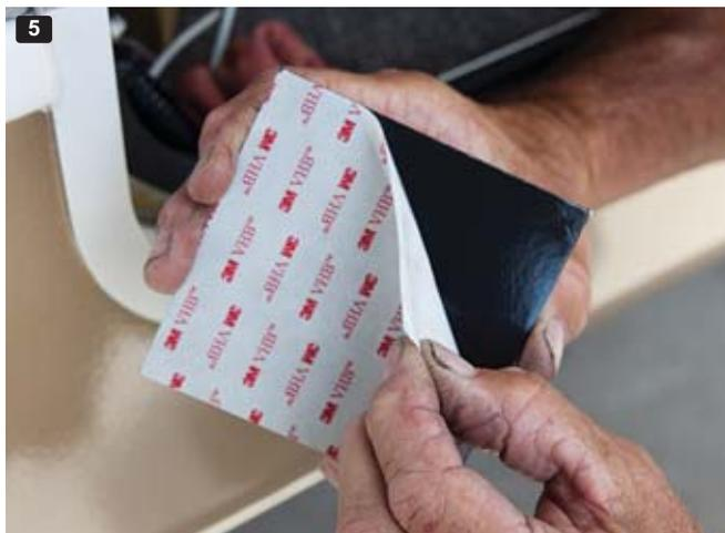
4) Next, follow the instructions provided and apply the primer to the roughed-up area. 5) Peel off the protective film on the mounting plate.
