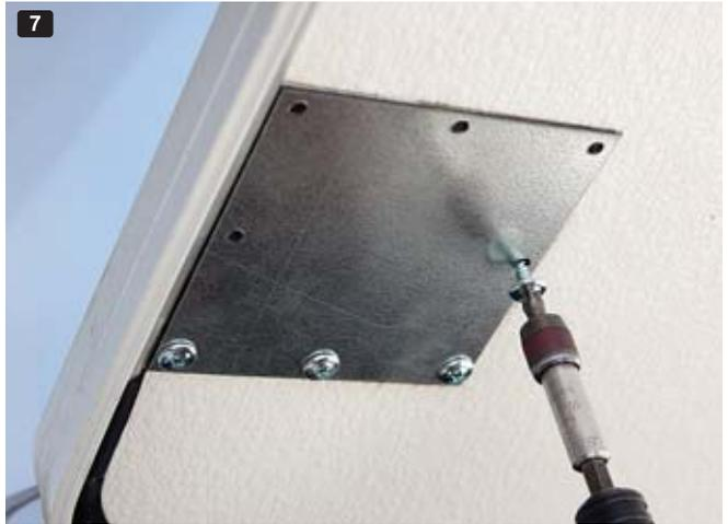
**6) Align the plate carefully, press and hold into place. 7) Using the provided self-tapping screws, drive the screws into place but do not tighten with a drill motor; you should hand tighten with a screwdriver to avoid stripping the screws or overtightening.**
