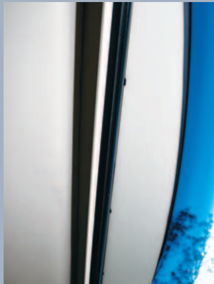
STEP 23. Next we snapped the new shade into place (according to the manual) with the shades turned in the correct direction to ensure the electrical motors can extend and retract the shades properly. Then we wired the power cords from the motors into the existing wiring for the coach. This allows the driver to open or close the shades from the cockpit. The wiring only consists of two power wires and two wires for programming the limit points. There is one wire that connects to a circuit that is only hot when the engine is running and this determines whether the shades have limited or full operation so they won't lower too far while on the road.
