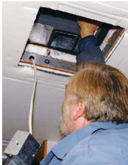
STEP 10. Now it's a simple matter of pushing up on the unit to break the seal. Typically, sealant isn't used at the factory, but the foam gasket can still get sticky with age.
