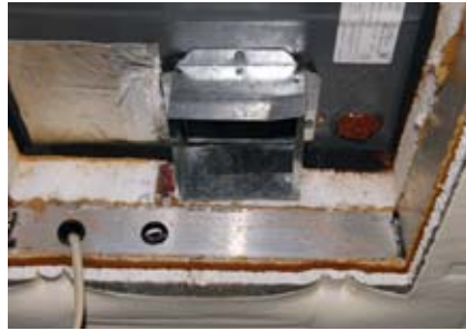
STEP 9. With the sheet metal removed, you can see the bottom of the A/C unit, along with the layers of block foam insulation in the roof.
