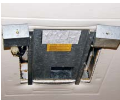
STEP 7. Next, the main cover is removed to reveal the sheet metal and ducting.
