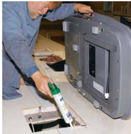
STEP 11. As mentioned, sealant is typically not used at the factory level, but Hall says a little bit provides extra insurance against leaks, especially on compromised surfaces. He centers the new unit over the hole, tips it back, applies the sealant, then carefully lowers the unit in place.
