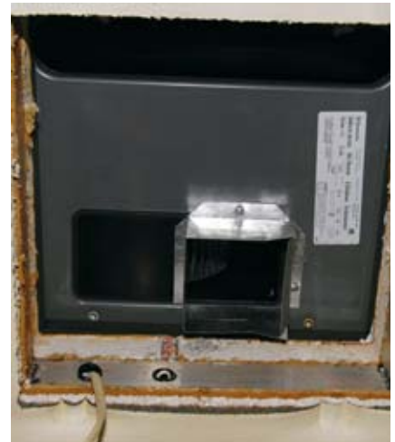
STEP 13. Once the unit is in place on the roof, go back inside the motorhome and make sure that it's properly aligned in the hole. If not, small adjustments can be made while the sealant is still wet.
