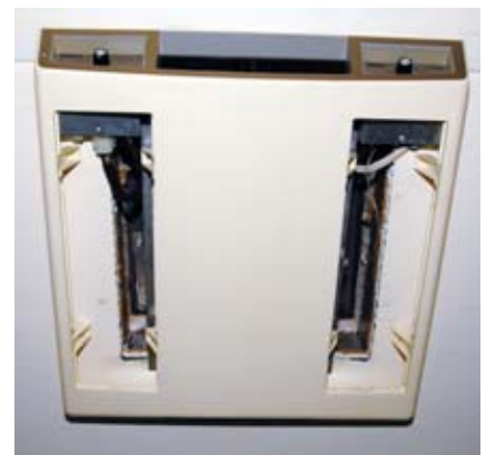
STEP 5. This unit had side vents that were removed to gain access to the main cover fasteners.
