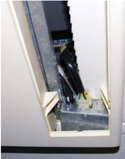
STEP 6. From this view, standing at the back of the coach and looking forward, you can see where the A/C unit's plug is connected to the power receptacle.
