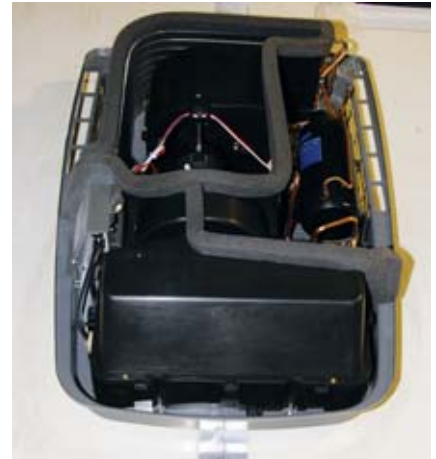
STEP 12. The new unit is now in place. Hall prefers to remove the cover before installation so it won't get dirty while being handled.
