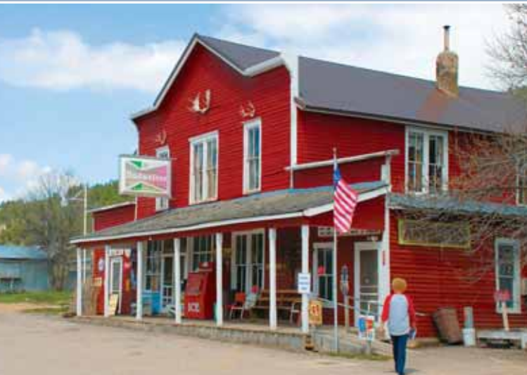
Aladdin General Store in Aladdin, Wyo., built in 1896, serves as the mercantile, post office and social center for the area. The store began as a saloon and commissary for coal miners.
