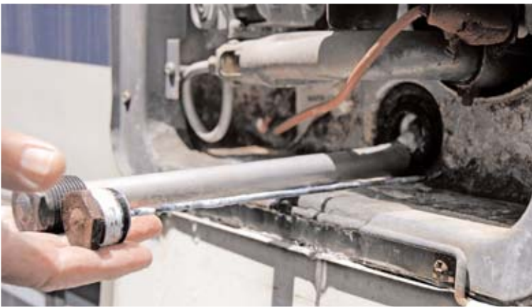
An anode rod should be replaced when material loss is at 75 percent. The old rod, right, is totally dissolved and well beyond time for replacement.
