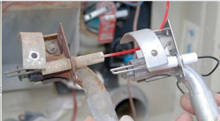
An old and new burner tube and igniter assembly.
