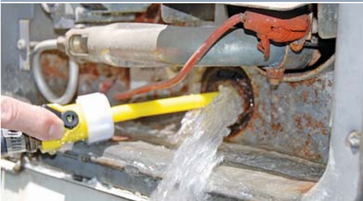
This convenient tool, which can be found at most RV stores, is used to flush the water heater. Periodic flushing is an important and easy maintenance procedure to eliminate minerals and other debris inside the tank.
