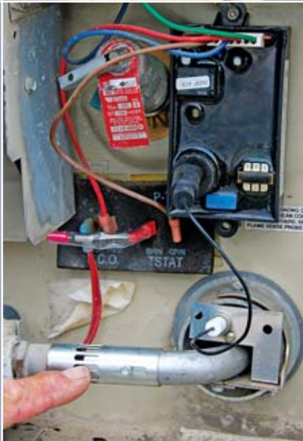
An old and new burner tube and igniter assembly.
