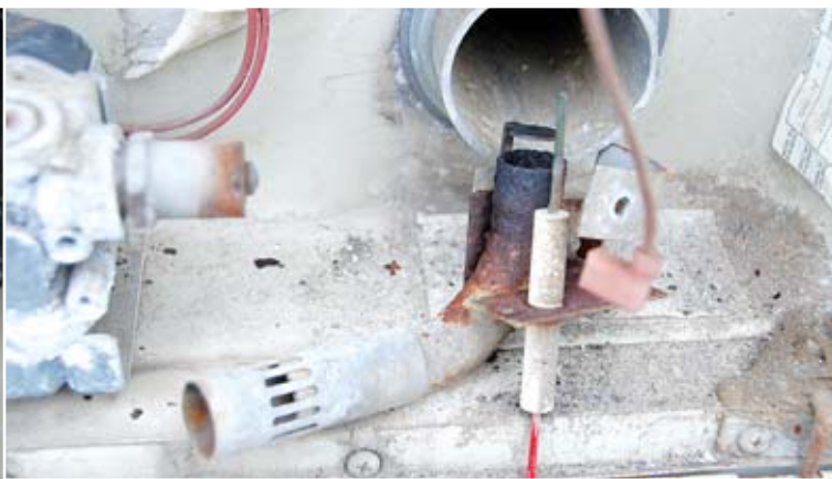
Rust on the burner tube can be removed with a wire brush or sandpaper before applying a coat of high-temperature spray paint. This water heater’s burner tube and igniter are beyond repair and need to be replaced.
