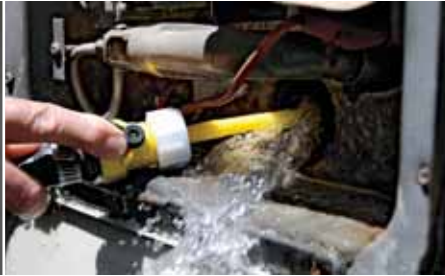
Drain and flush the water heater using a water hose attachment.
