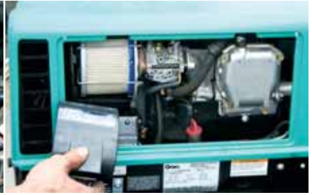
Generators should get regular oil and filter changes as well as tuneups.
