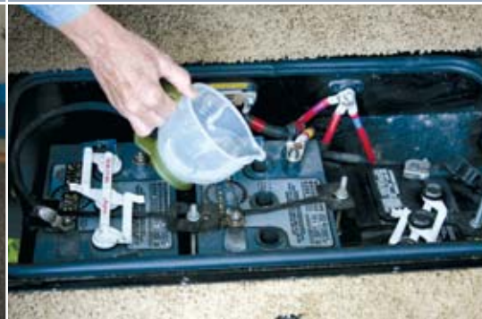
Batteries should be at full charge, with electrolyte filled to proper level using distilled water.
