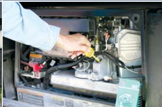
As is the case with motorhome engines, an ideal time to change oil and filter in an AC generator is shortly before winter lay-up.
