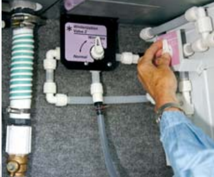
In this coach, antifreeze valve and water heater bypass, right, are side by side.
