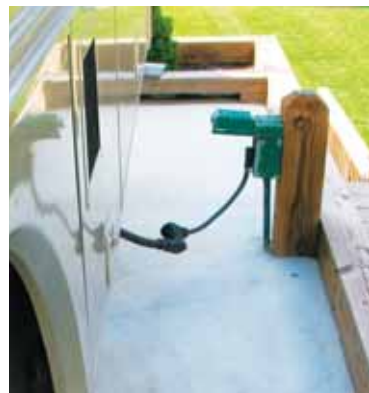
Our parking pad includes a 30-amp hookup, which connects to the electrical panel in our basement.
