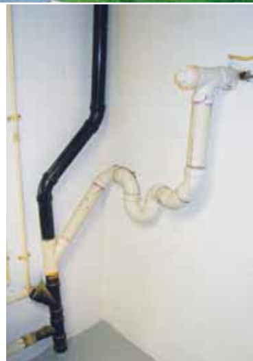
During construction of our home pad, a plumber hooked up piping to our existing sewage system.
