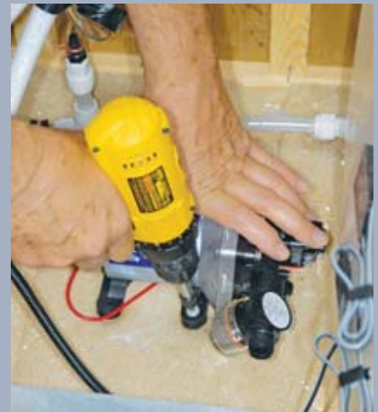
The pump base grommets should not be over tightened, but snug enough to keep it from breaking loose from its mounting surface.
