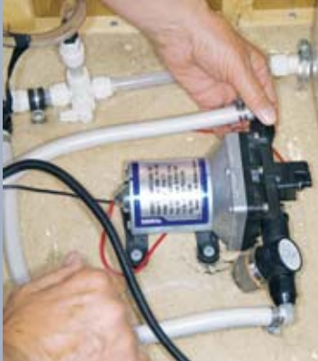
If the pump is cycling with all of the faucets closed, check the inlet and outlet for leaks
