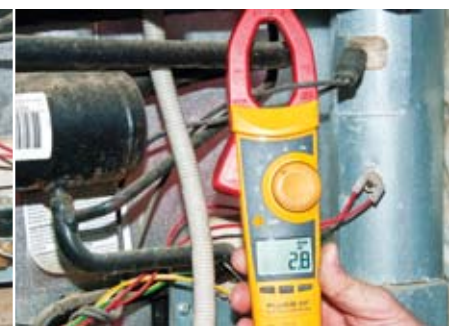
Clamp meters provide a quick and easy way to verify the refrigerator element is working.
