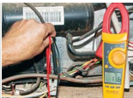
Always check directly at the appliance for voltage to controls and components. Acceptable ranges are referenced in service manuals.
