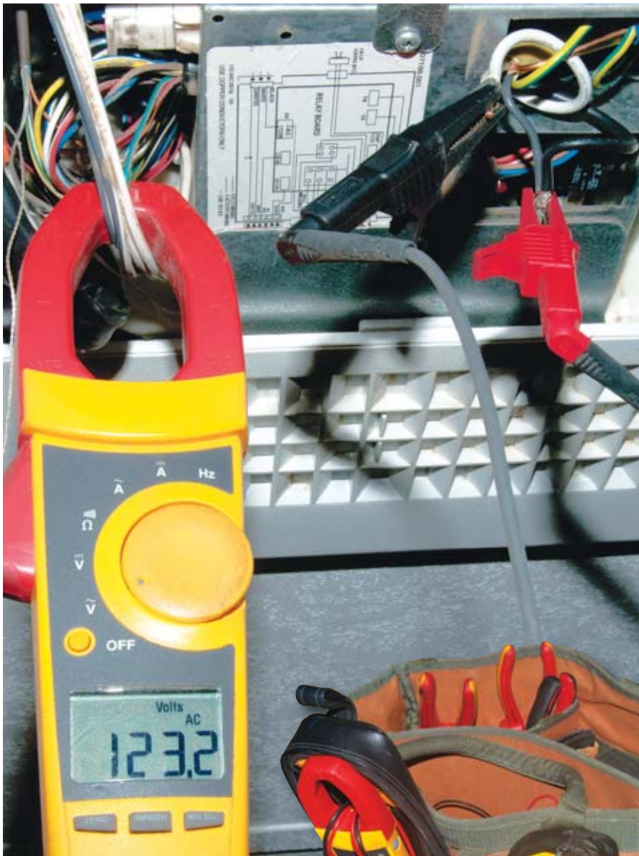
Using a meter to verify voltage at the air conditioner. The acceptable range is 104-132 volts AC.
