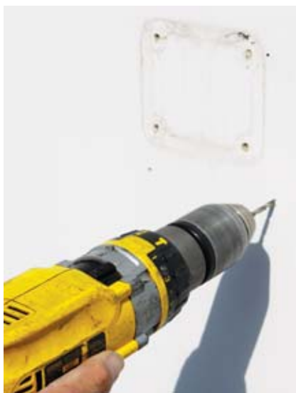
3. Once the holes have been marked, pre-drill with the proper-size drill bit.
