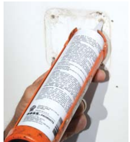
5. Apply silicone sealant to the old and new holes to ensure waterproofing.
