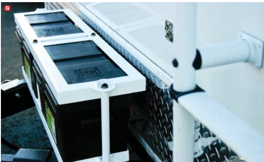
G) The final product neatly sits on the trailer's A-frame and the batteries have maximum protection from the elements — and unauthorized hands.
