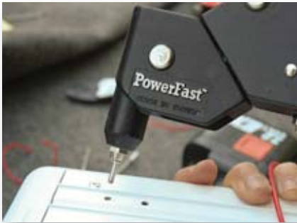
7) We used a PowerFast pop-rivet gun to reattach the ballast cover, making sure it is secured.
