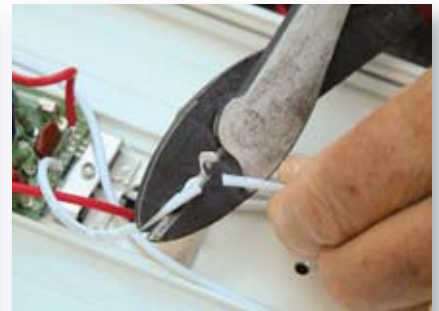
2) We cut the ground wire from the ballast to the switch.
