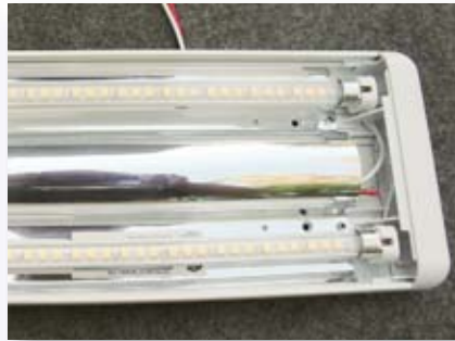
8) Star Lights were a direct replacement for the original compact fluorescent tubes.
