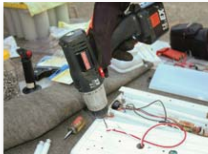
1) The ballasts covers on our Optronics were attached with small pop-rivets that needed to be drilled out.
