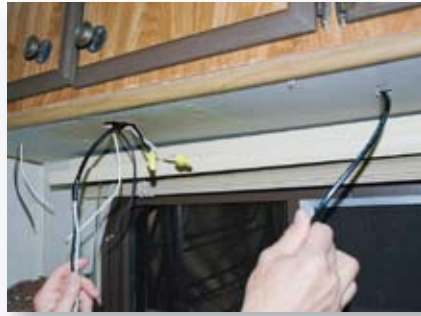
10) A "snake" was used to feed wires to the new Optronics reading lights.
