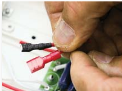
3) We reused the small quick-connect from the Optronics wiring. Star Lights supplies quick-connects, but they are larger.
