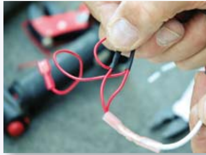
6) The Star Lights harness wires were spliced into the Optronics negative and positive switch wires.
