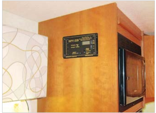
Mounting the Heliotrope charge controller next to the RV's doorway was a good idea, as it made it easy to keep an eye on battery conditions frequently.
